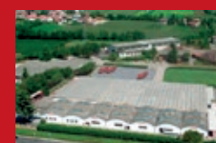
Trainign center, produzione scambiatori radianti Training center, production of radiant heat exchangers Via Sile, 17
